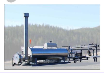
Figure 2— Indirect-Fired Line Heater at Wellsite (*Courtesy of Presson* ENERFLEX and Petro-Canada)
