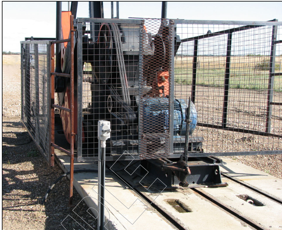
Figure 6 —Steel Skid Bolted to Base
